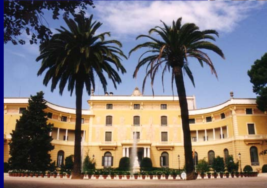
(Pedralbes Palace, official Secretariat's building)
